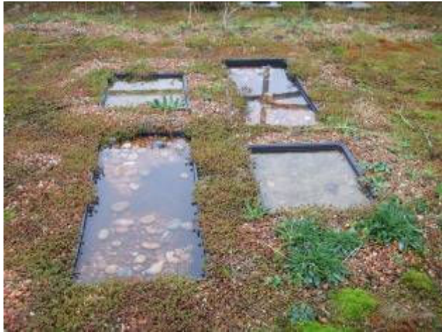
Green roof with water feature
